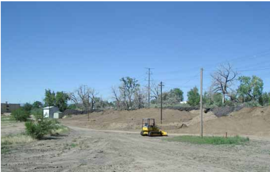
Grading and compacting of community soils
